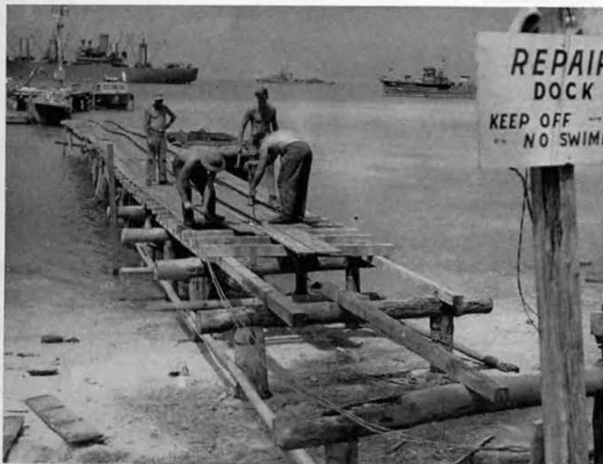
This close-up shows the poor workmanship of the Japs.
