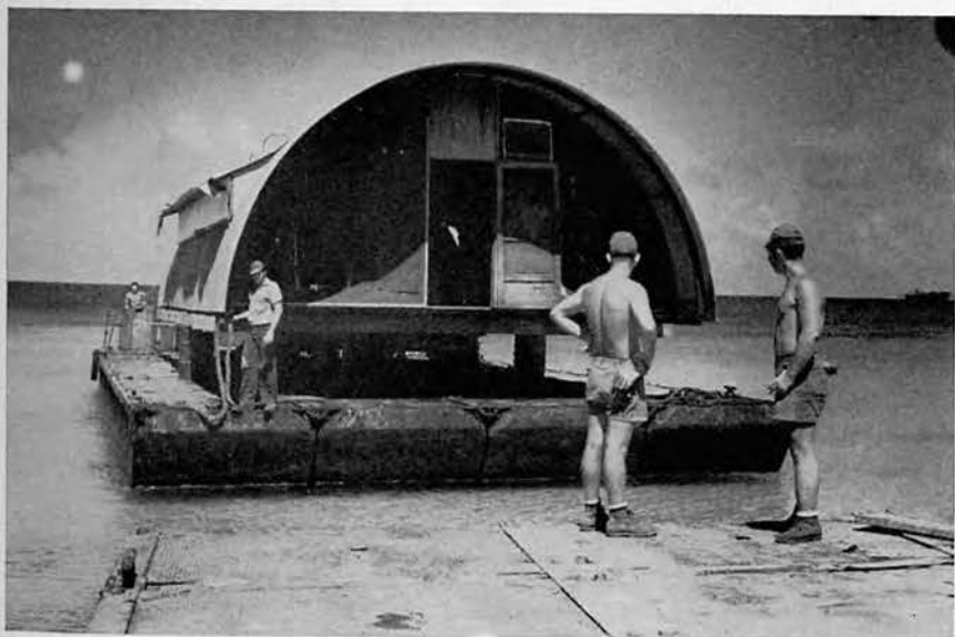
The floating hut arrives at the dock.
