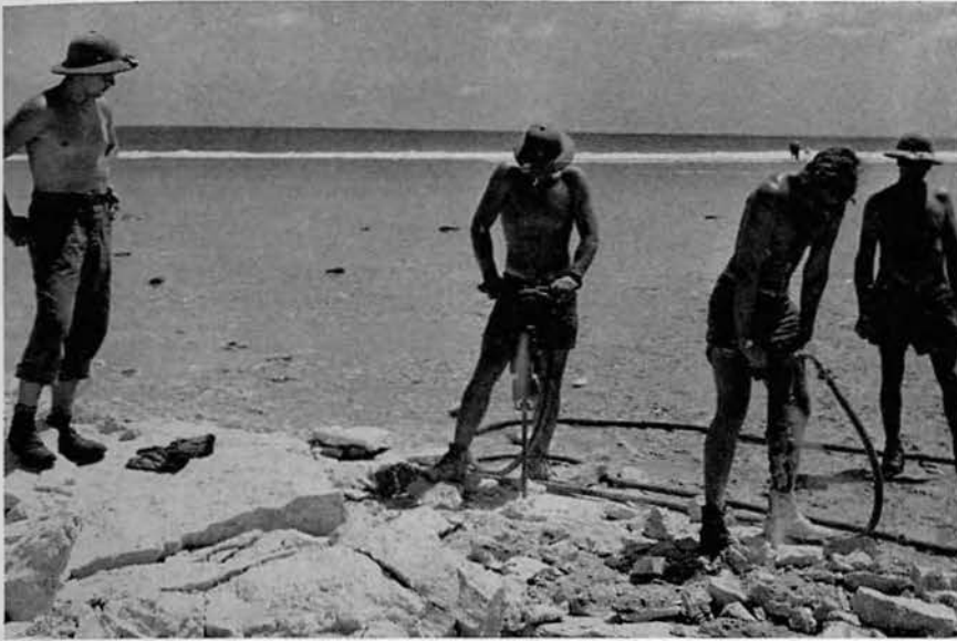
Air hammers are used to break the hard coral.
