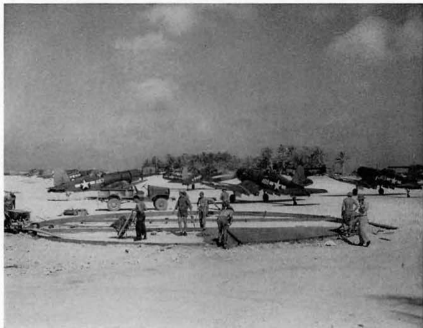
Like a huge pie, the sections are poured while planes come and go.
