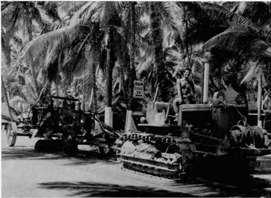
The heavy, daily traffic found our main road in first class condition. Thanks to this team.
