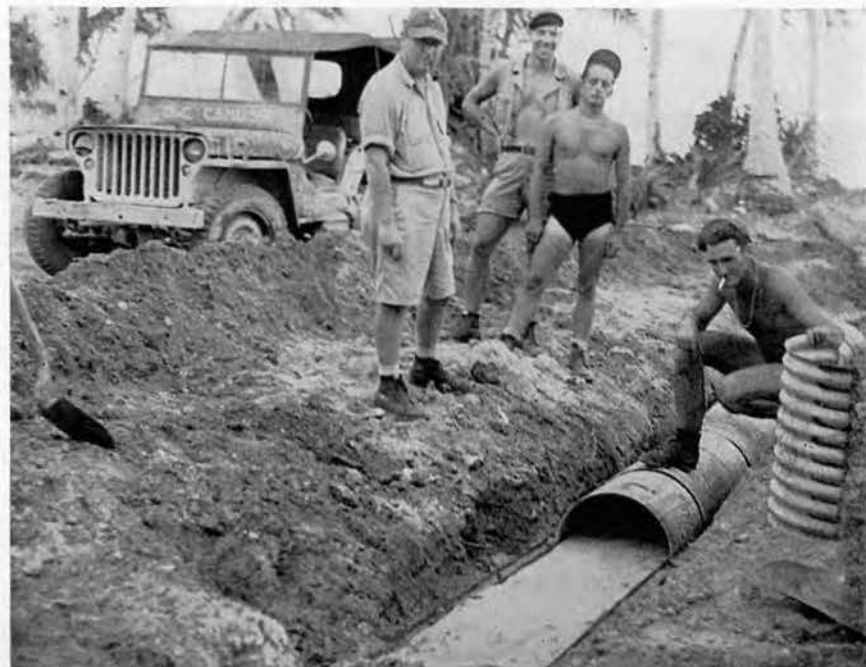
Drainage of areas was a hard but very necessary job.
