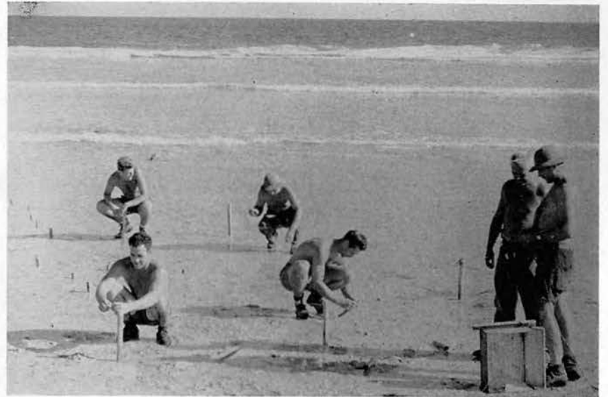
The charges are carefully set and fused.
