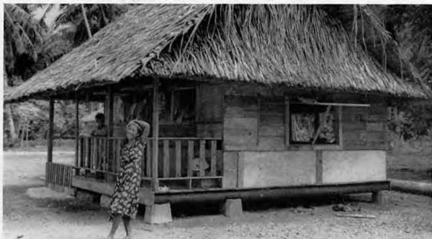
Built by natives, construction influenced by American ideas.
