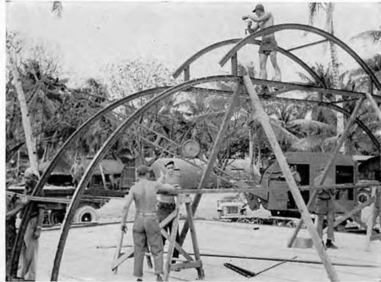
No. 2 in place. It won't be long now.
