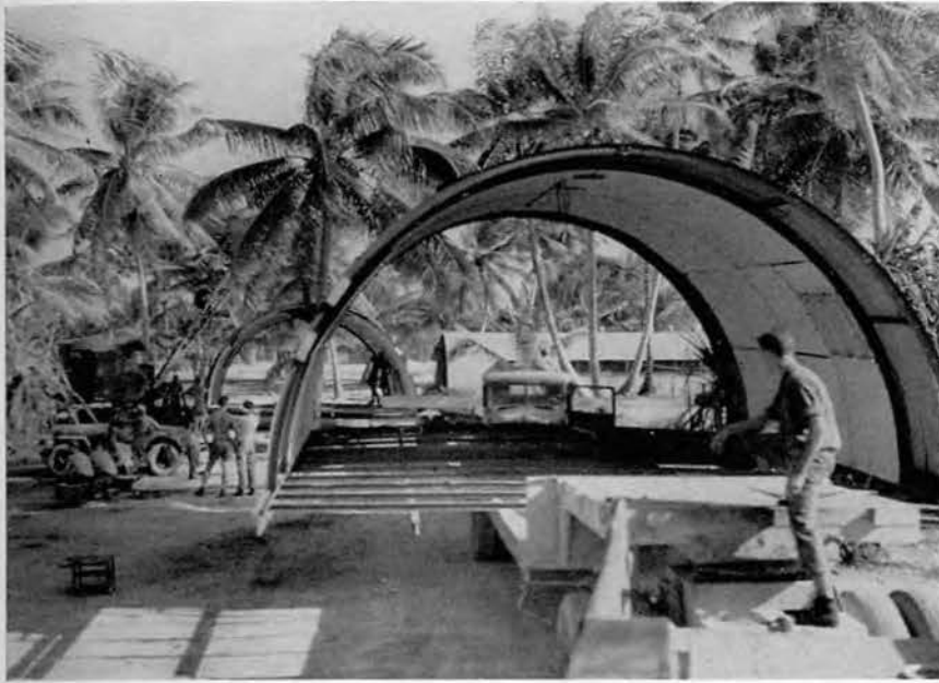
Quonsets are cut in two and loaded on trailers.
