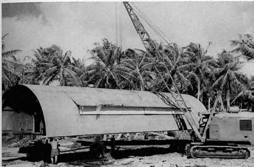
In one piece it's lifted and set on the trailer.
