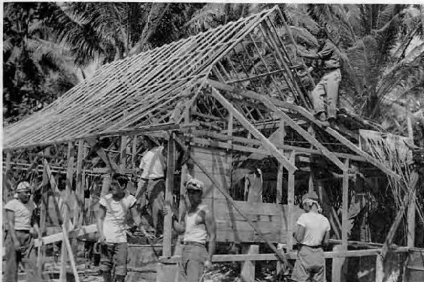
A new home under construction.
