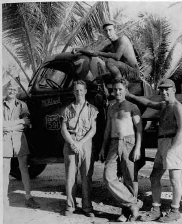
The barge and pile driving crew.
