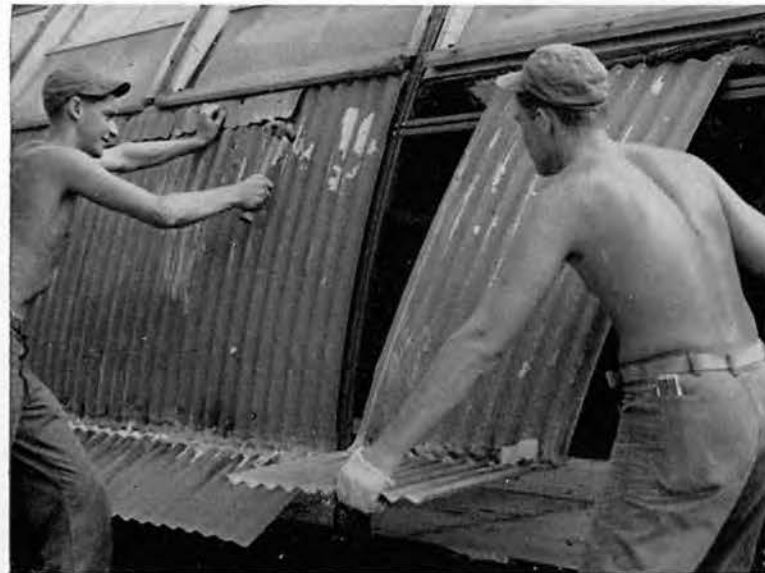
The re-shaped sides go into place as though made to order.
