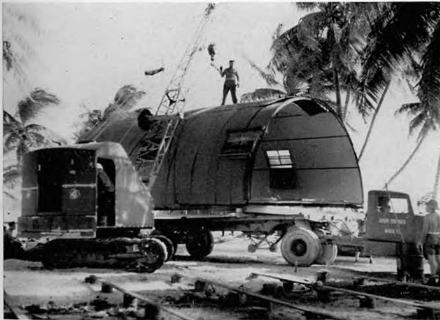
Using larger trailers, a hut is lifted intact and ready to move.
