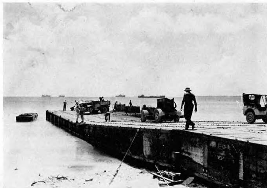
Docks were in constant need of welding experts.
