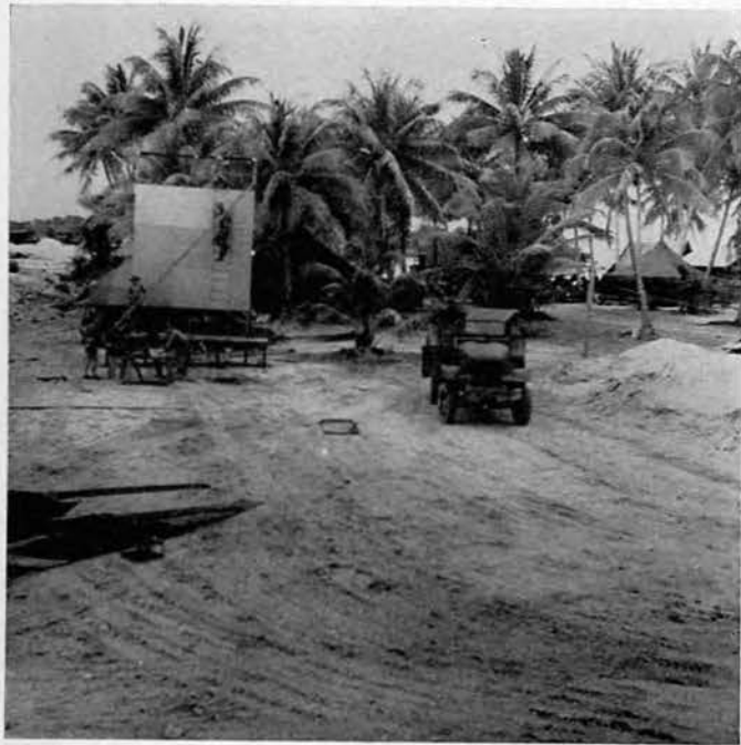
Grading the area and building the screen at the same time.
