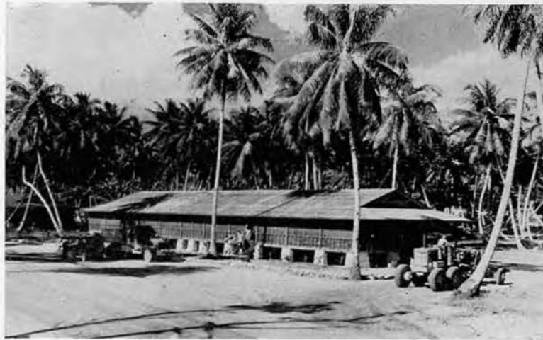
Jap building now used as a Fleet Post Office.
