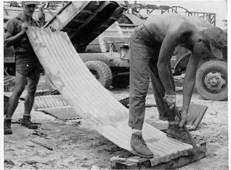
The galvanized sides are shaped to fit the new design.
