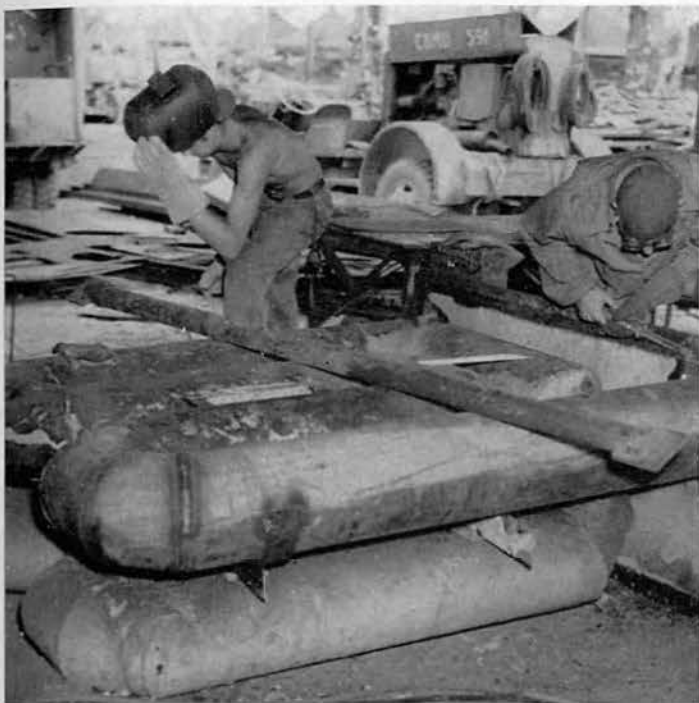
Working on part of water distillation unit.
