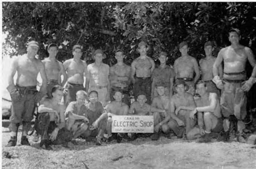
Electrical Maintenance Crew.
