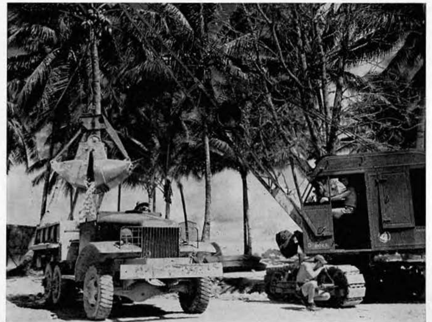
We dig a sump and the coral is used in other places.
