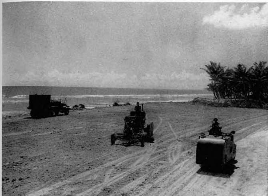
Heavy equipment men making new parking area.
