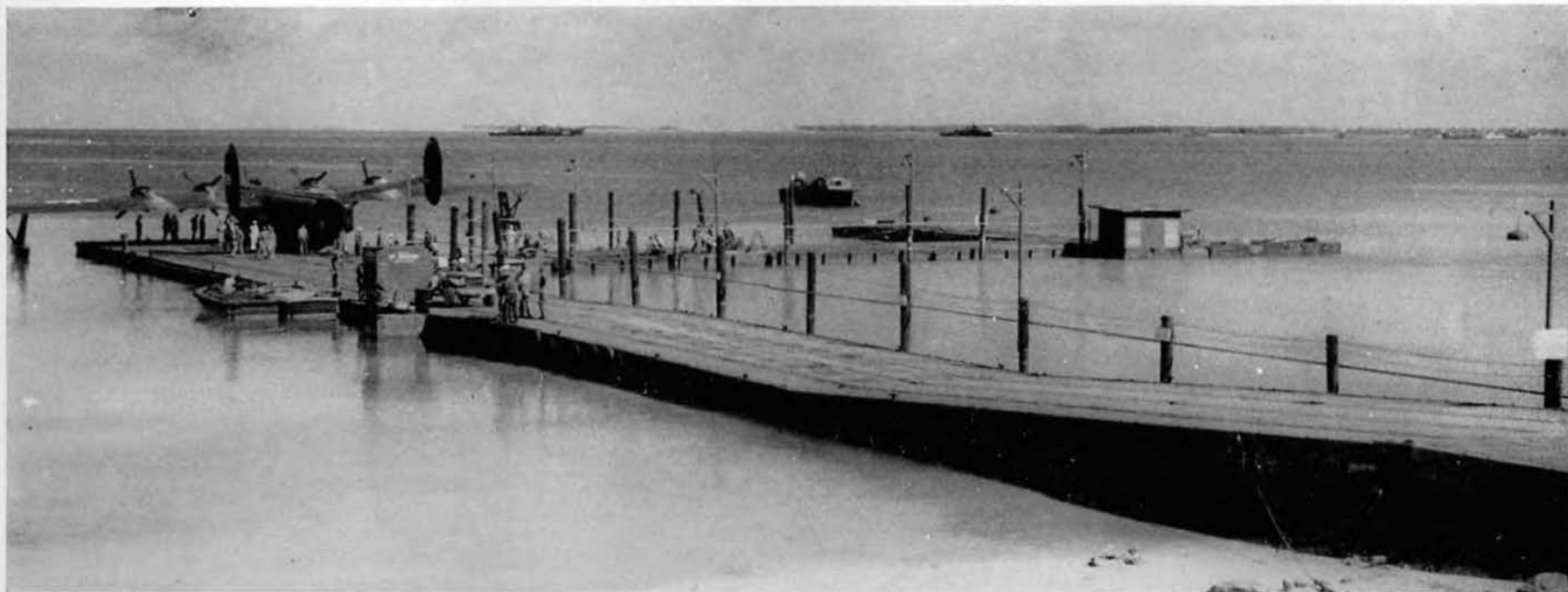
The completed dock, where transients, supplies, and mail, will be but a day or so from home.
