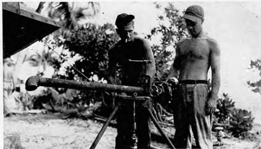
Cutting pipe is a man size job.
