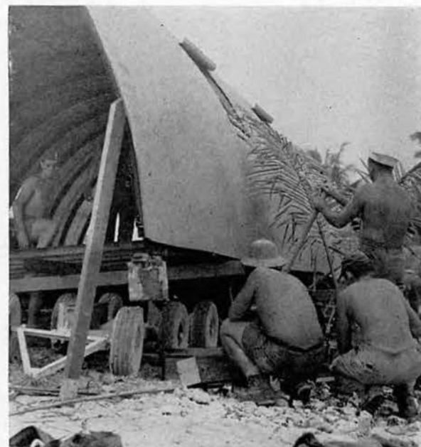
The dollies in place the hut is lowered.
