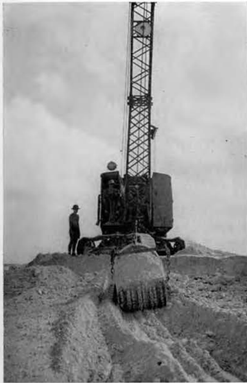
A dragline at work.
