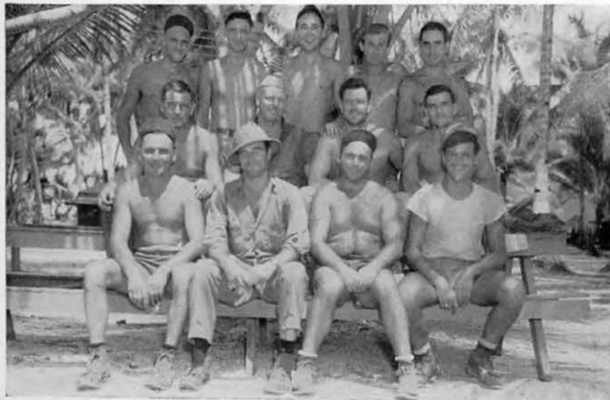
Structural carpenter gang.
