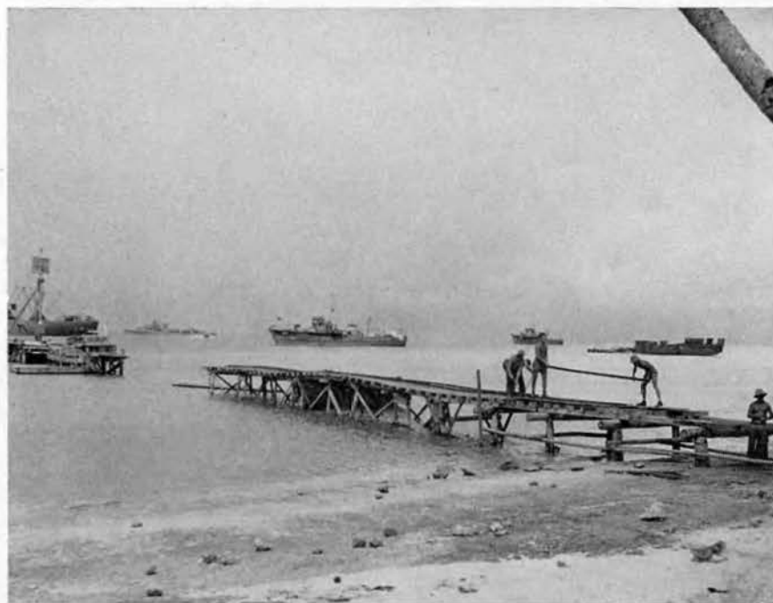
Practically falling apart, we make a complete job of dismantling.
