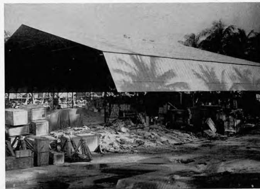
Corrugated roof finishes the job.
