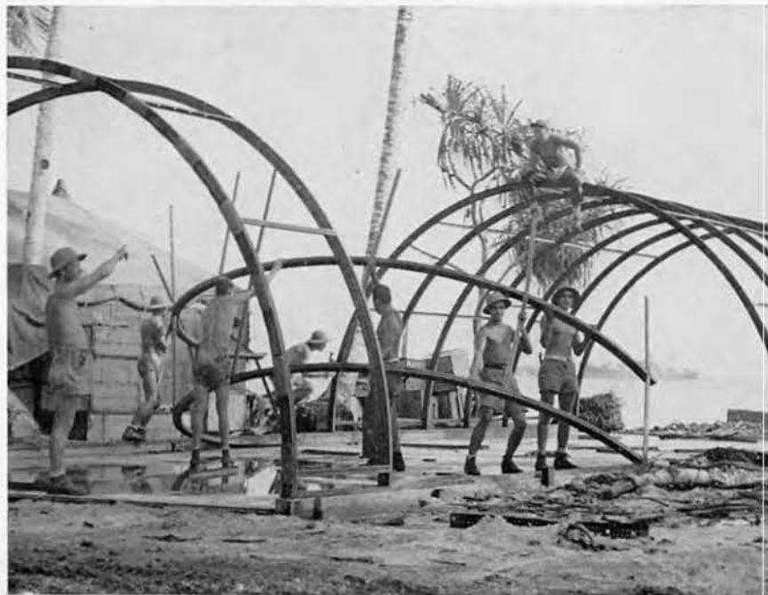
The ribs are easily fitted into place by those who know how.
