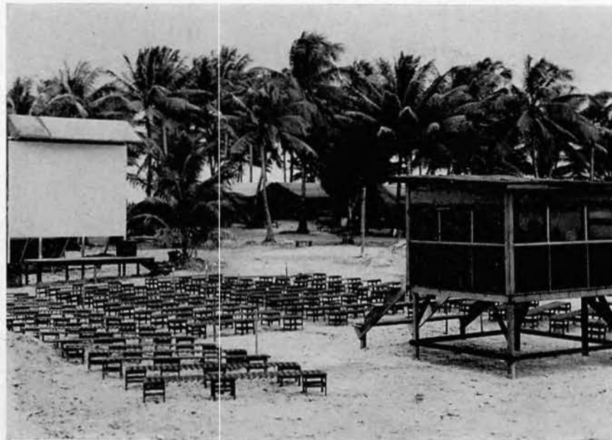
Completed. On with the show.
