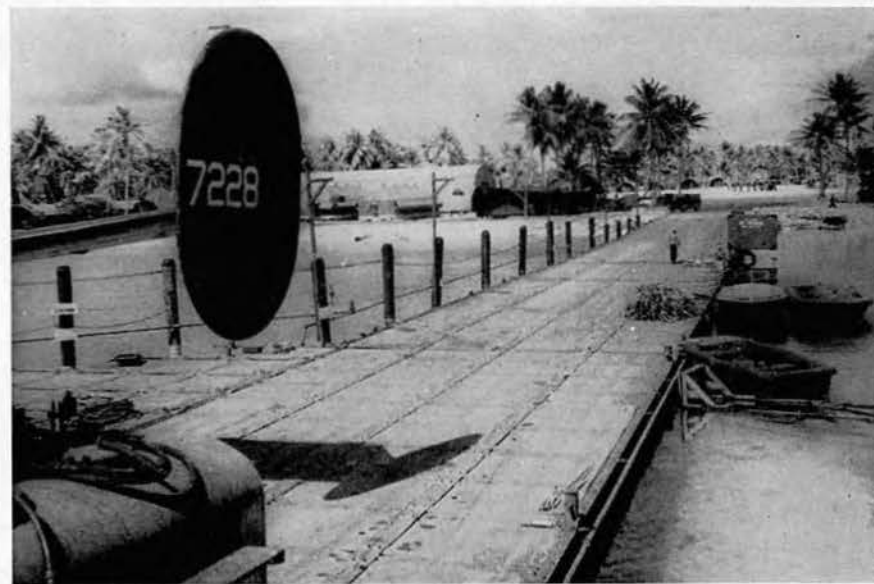
The completely assembled dock shows how well the men did their job.
