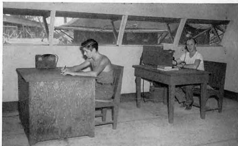
Interior of Office. Zampieri, Messenger, Corey, Jr. O.O.D., on the switchboard.
