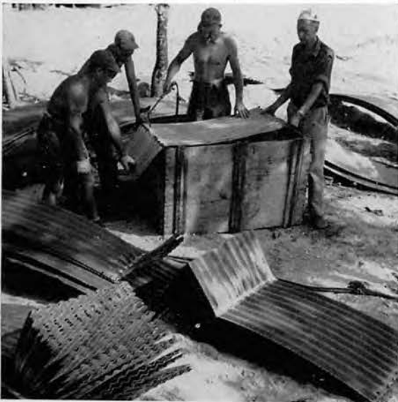
Heat is applied to make the corrugated steel pliable.
