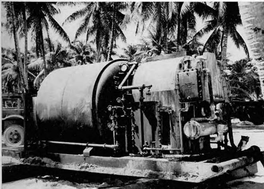
Job partially done.
