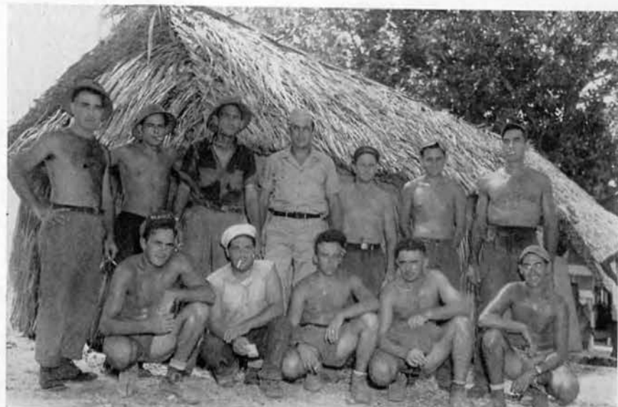
Carpenter and cement finishing gang.
