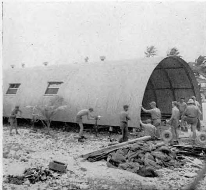
One side at a time, the hut is jacked up.
