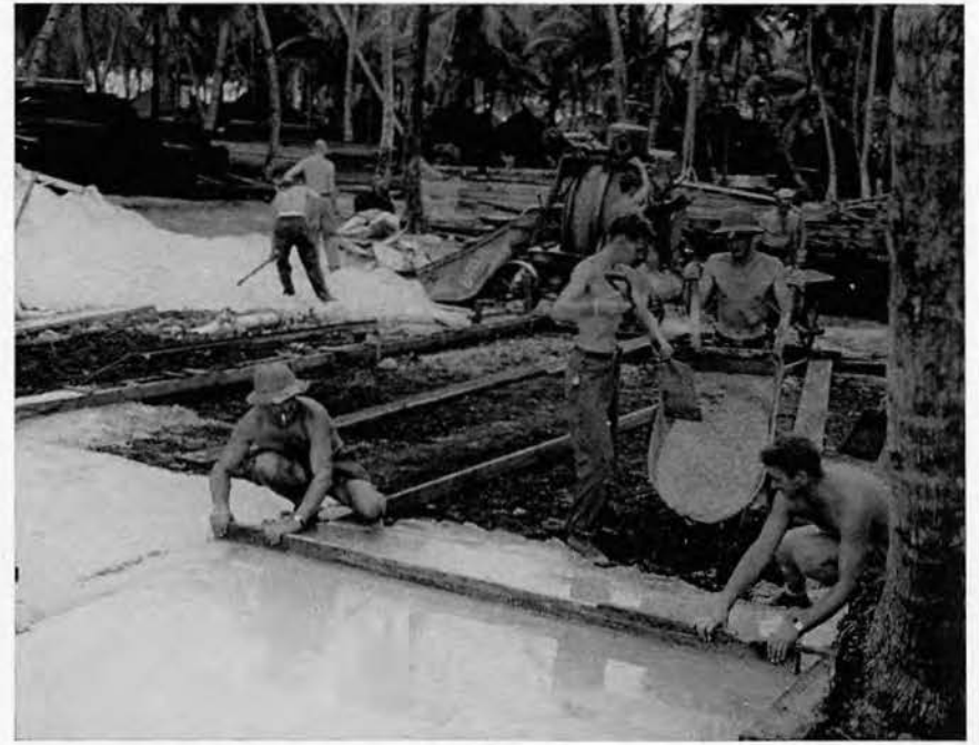
Concrete is poured and finished, making a good foundation.
