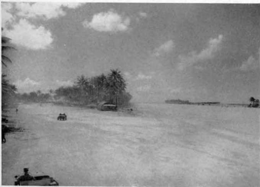
Taxiway looking towards the air strip.
