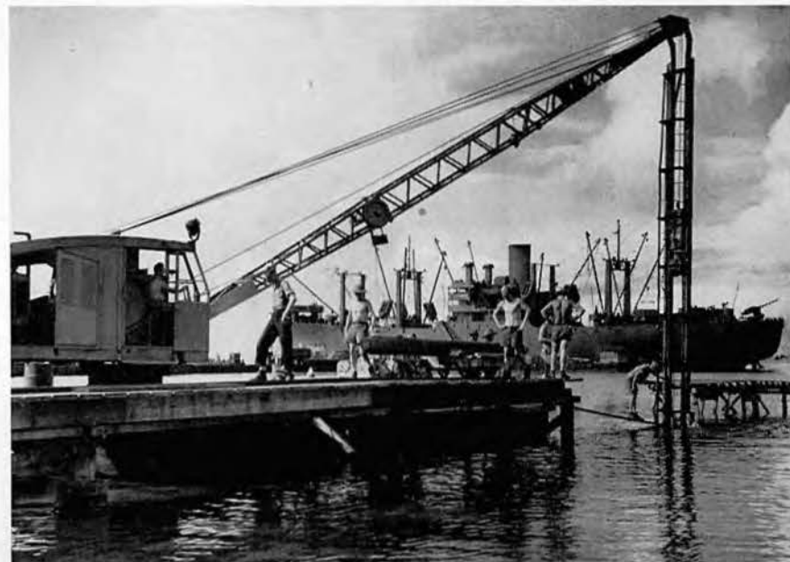
The hammer is set to drive one.
