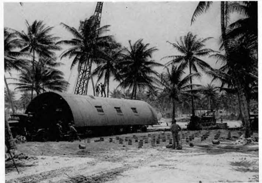
At the new location the site is ready when the hut arrives.
