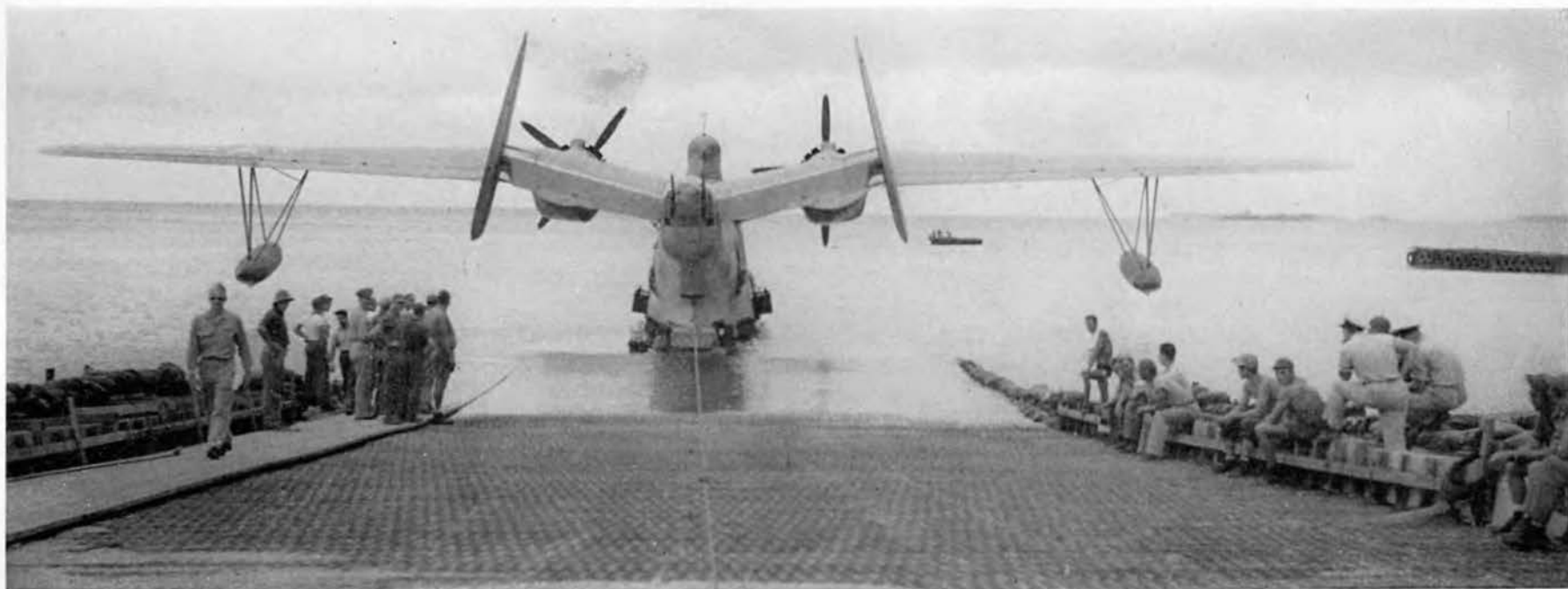
The first plane is beached and the ramp is officially open for business.
