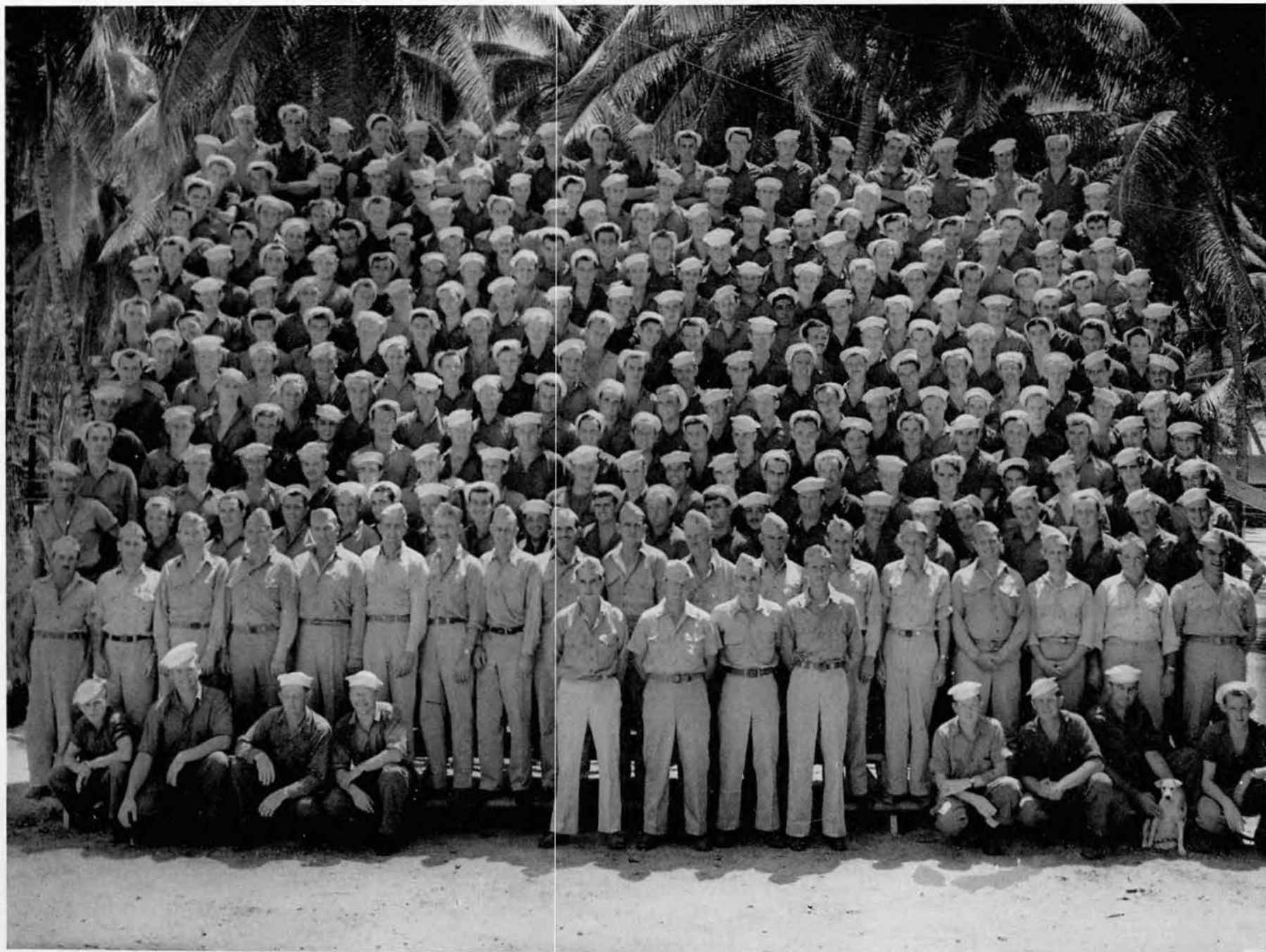
Construction Battalion Maintenance Unit 591 Majuro Atoll—May 1945
