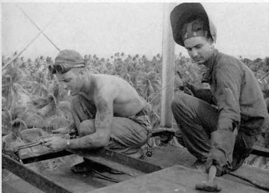
Repairs needed at 110 feet in the air never stopped the welders.
