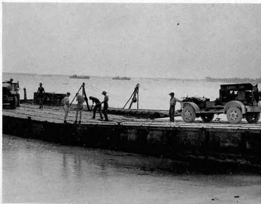
Portable welding units move on the scene.
