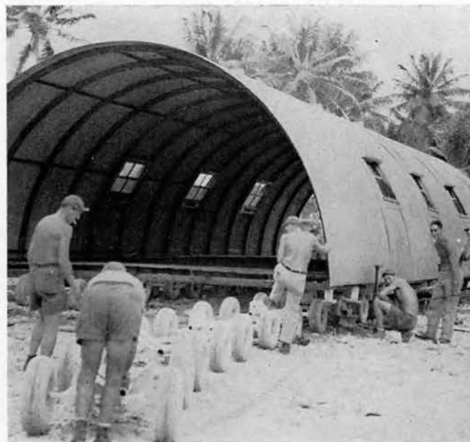
A bomb dolly trailer is rolled under one side of the hut.
