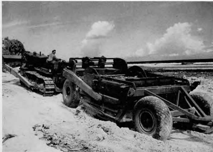
Dirt is easily hauled and spread with a "carry-all".
