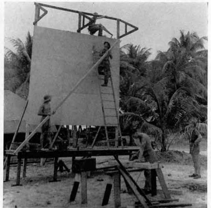
2 x 4's and sheets of plywood make an ideal screen.
