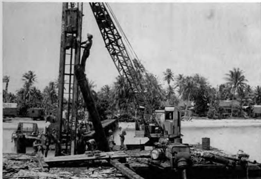
Up goes the hammer and the piling is placed.
