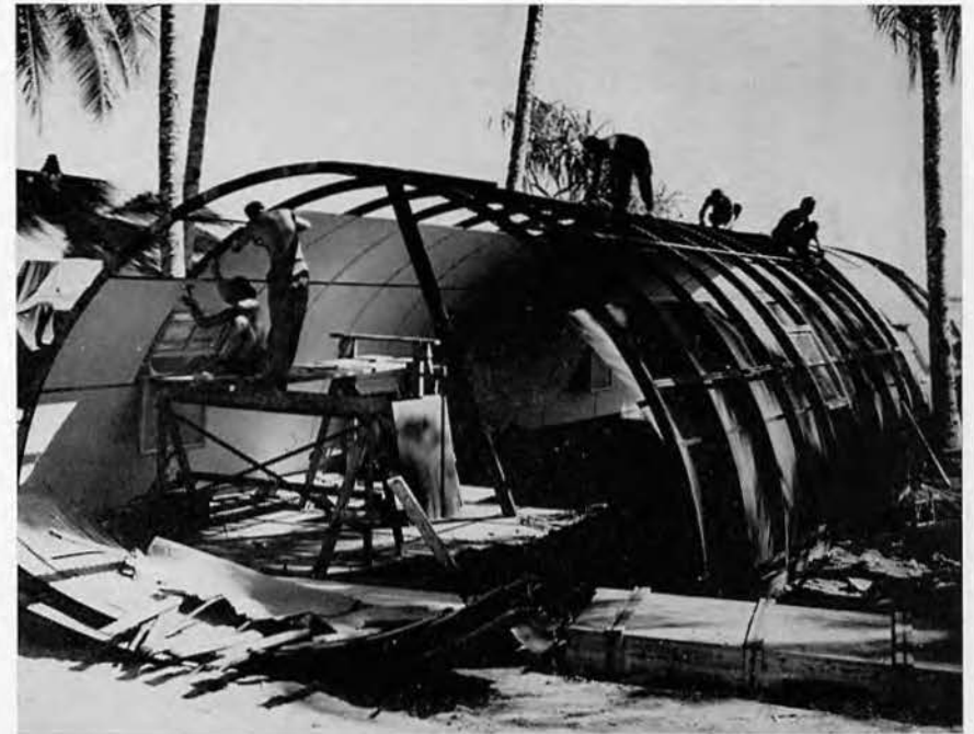
The insulation and wall boards find their place.
