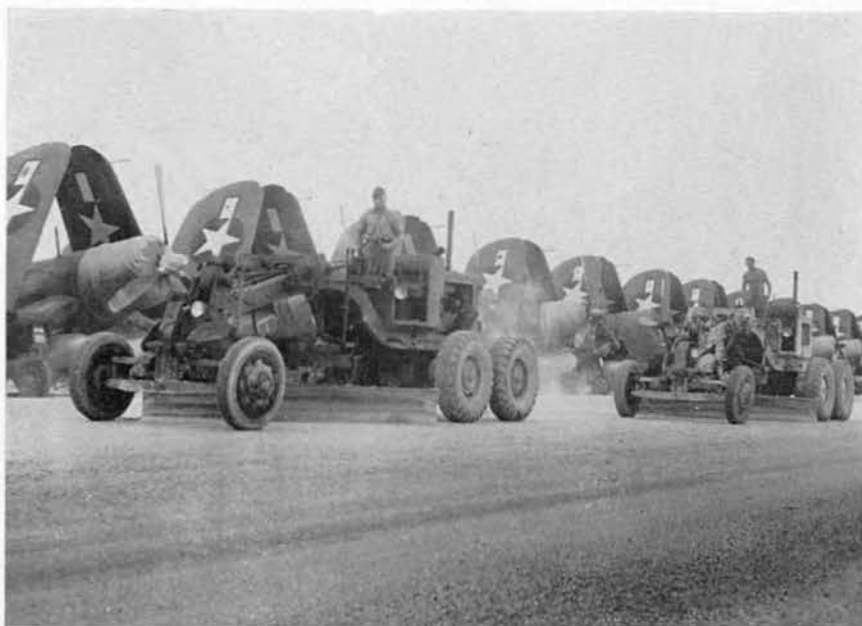
Parking area is kept in good shape.
