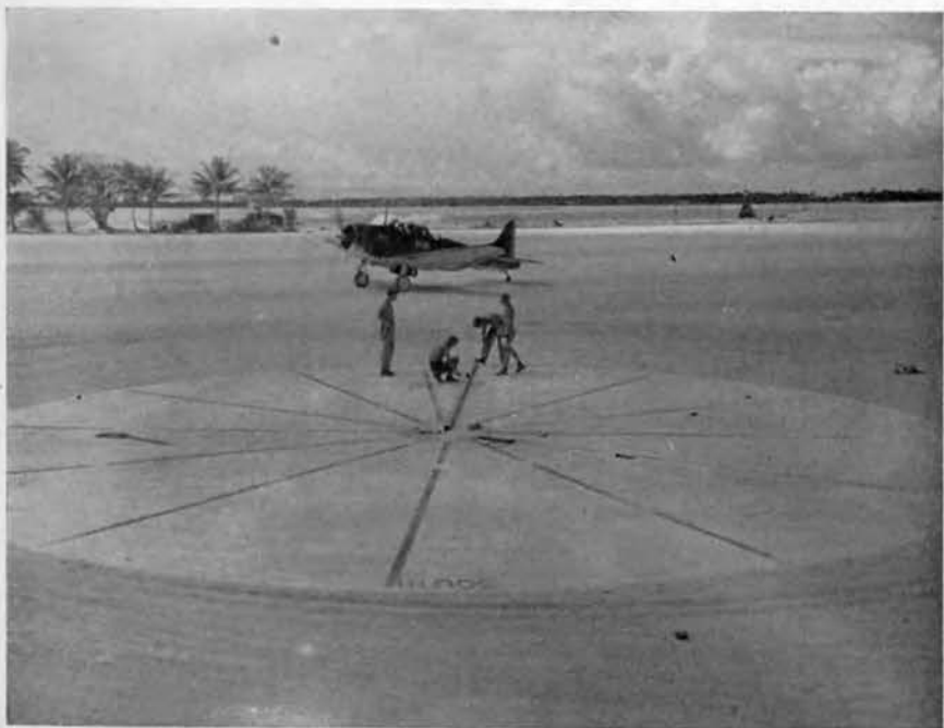
The surveyors check the points of the compass as a plane stands by.
