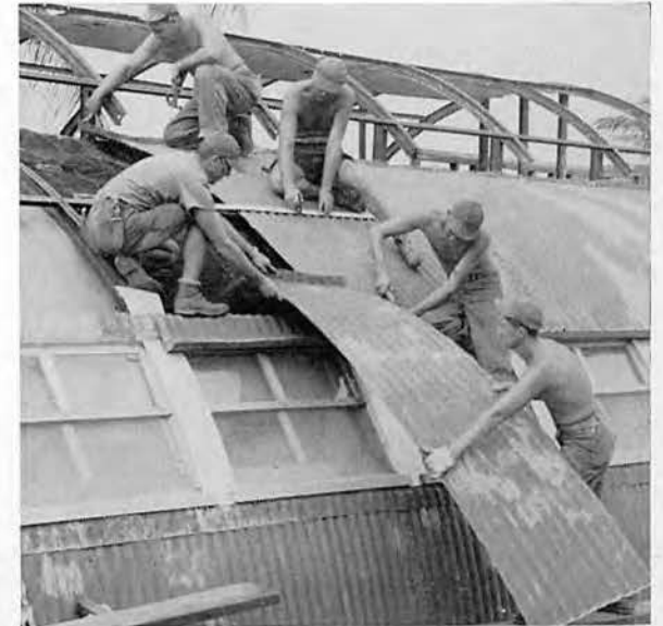
The windows are in, now for the roof.
