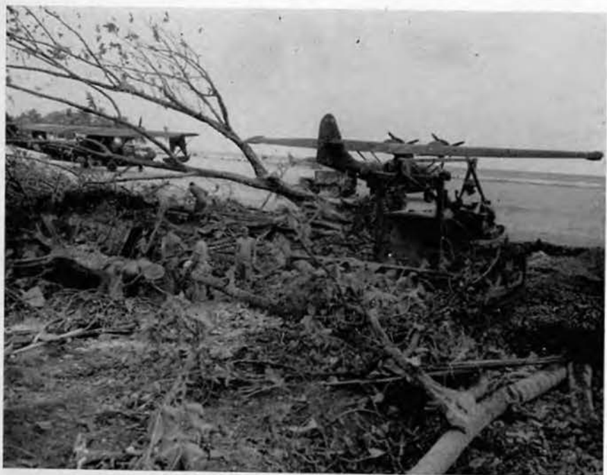
Removing debris for construction of hardstands for PBV's.
