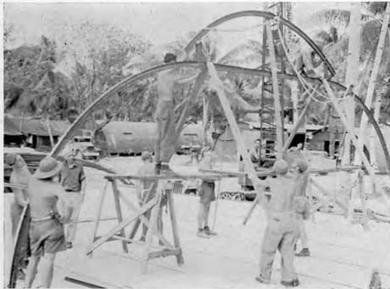
The first rib swings into place and is quickly braced.
