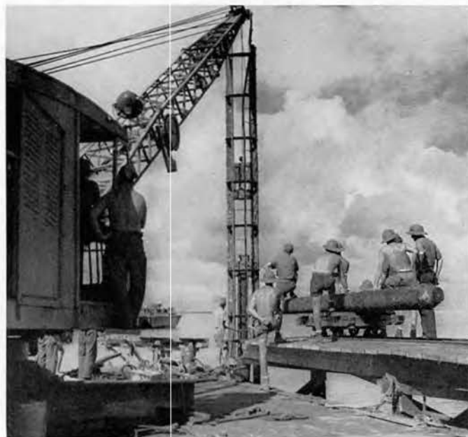
Pile driving rig mounted on a pontoon barge.
