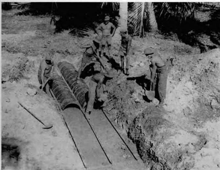
Old oil drums were salvaged and used as culverts.
