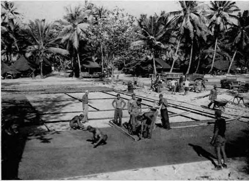
Our first concrete tennis court under construction.
