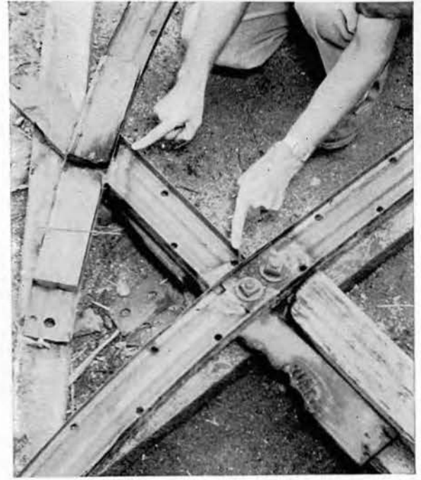
The rib extensions in place, and a tropical top, in two welds.
