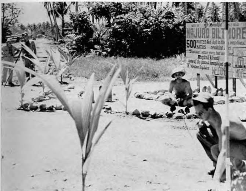
Surveyors staking a position for road drainage.
