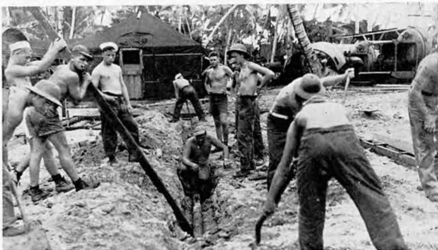
The plumbers dug their own ditches.
