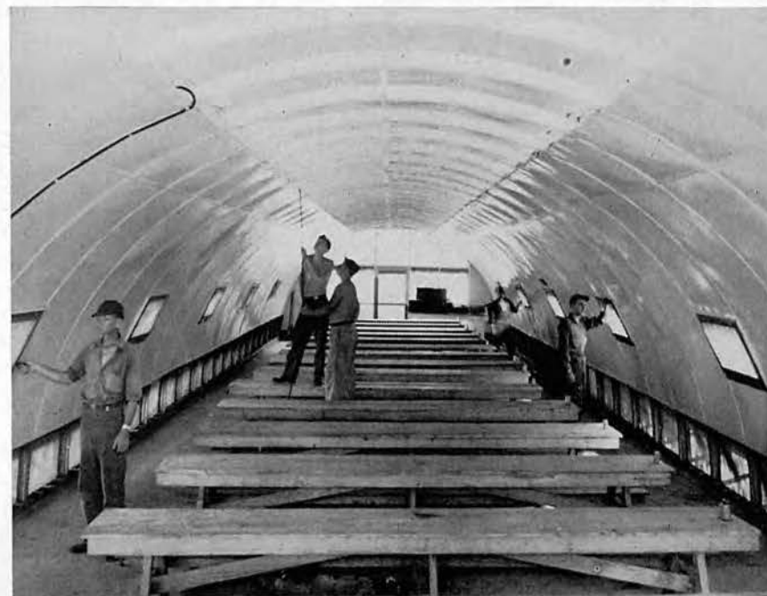
Completed in record time. Paint gang and electricians finishing their job.
